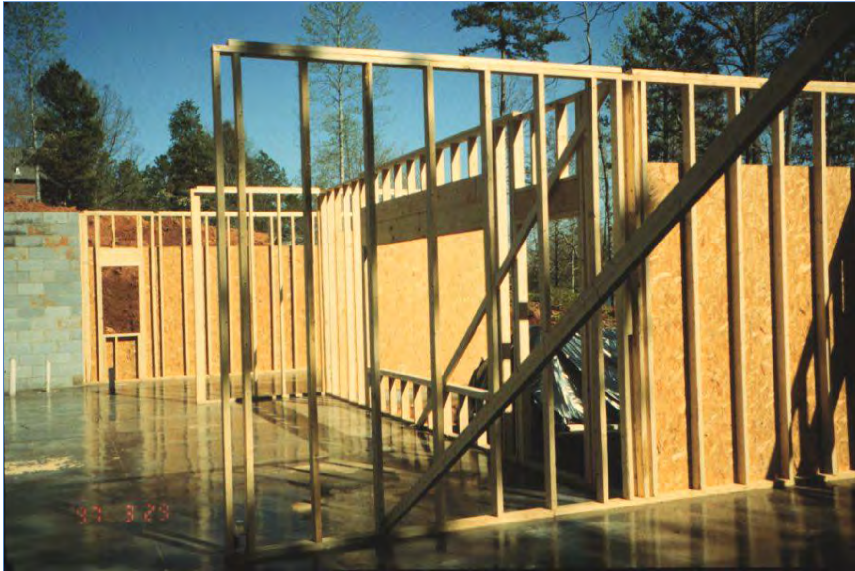
LIGHT WOOD FRAMING: Balloon e Platform frame
