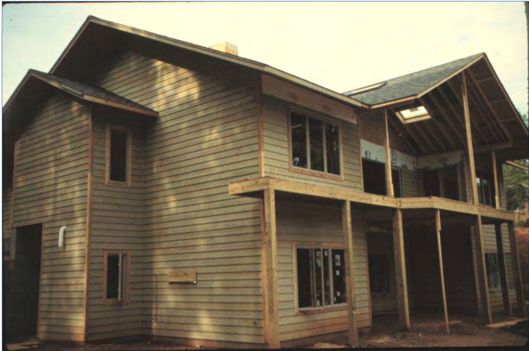
LIGHT WOOD FRAMING: Balloon e Platform frame
