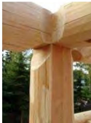
Raccordo Pilastro - Architrave
